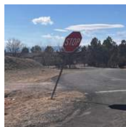
Stop sign POST broken off
