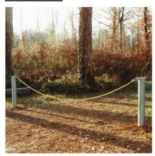
A bollard or fence would be placed on either side of the road and a chain would be strung across the road. The system could have break away capabilities so that, in the event of a collision, the chain would break to minimize the damage to the impacting vehicle.
