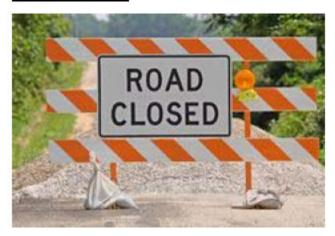
A Type III Barrier is a common traffic control device used to close roads. Type III Barriers are not attached to the road and typically weighed down by sand bags.
